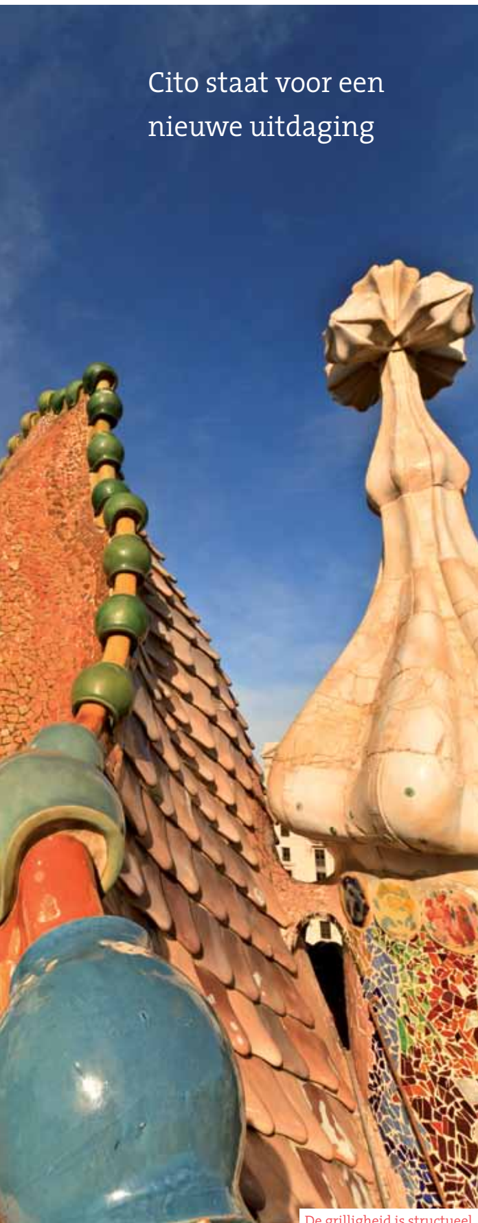
De grilligheid is structureel.
